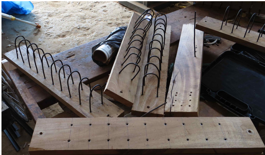
Figure 4.6: Planks in various states of installation.
